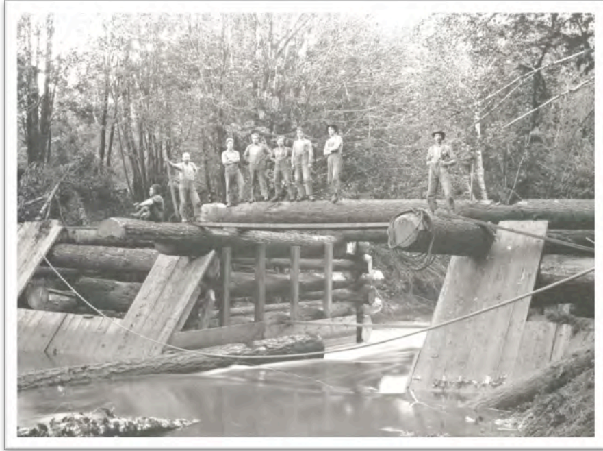
Photo 1: Assen Brothers Splash Dam in 1912, Middle Creek Oregon. Photo courtesy of Coos County Historical Society
